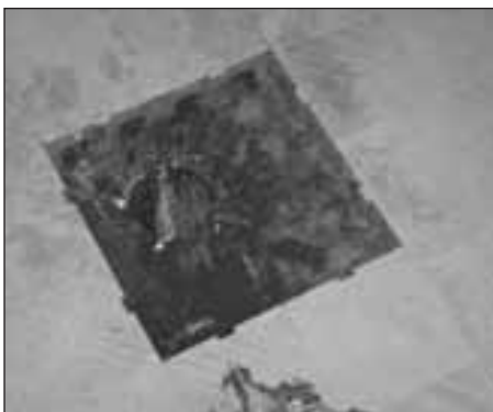
Removed tile showing under drain tile
