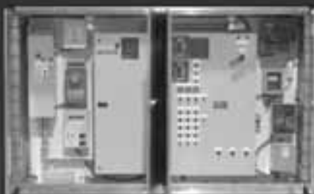
Pad Mounted Control Packages
