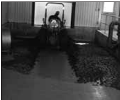
Dan removing sludge from Filter Bed
