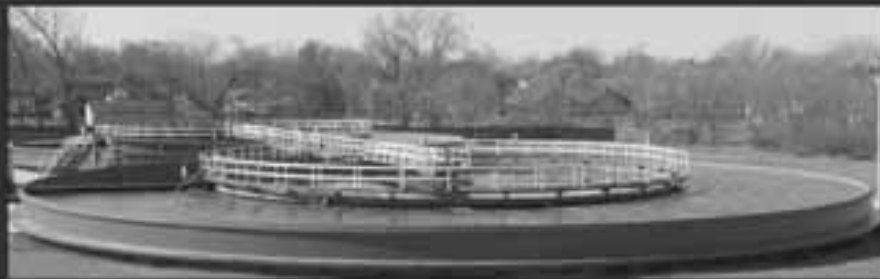
Wastewater Treatment Solutions
